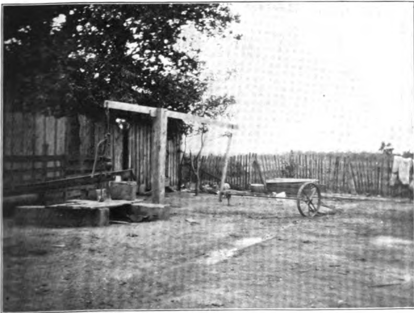
B. APPARATUS FOR PUMPING BY HORSEPOWER.
